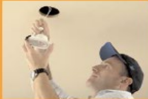
Downlight removed and supply disconnected
