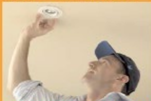
Downlight reconnected and fitted as normal with transformer outside the cover
