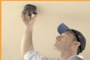
Cover fed through downlight cut-out
