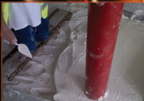
Trowelling up the Intucompound Seal
